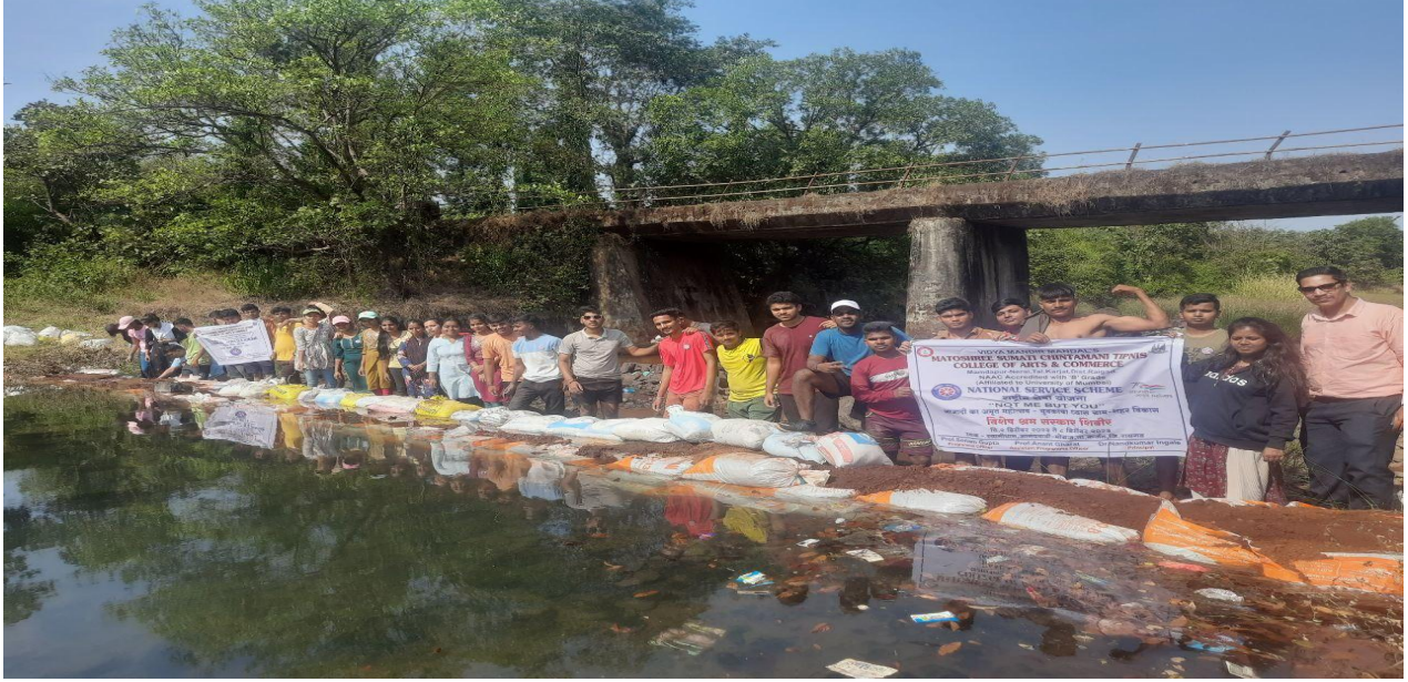
Construction of a bund on the river in Anandwadi village
